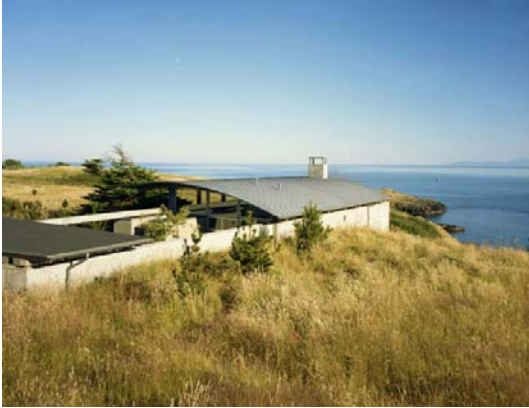
American Camp, a residential project on the Pacific Ocean, has a vaulted roof shell covered in battens made of zinc. Photo by Paul Warchol, courtesy of Suyama Peterson Deguchi
